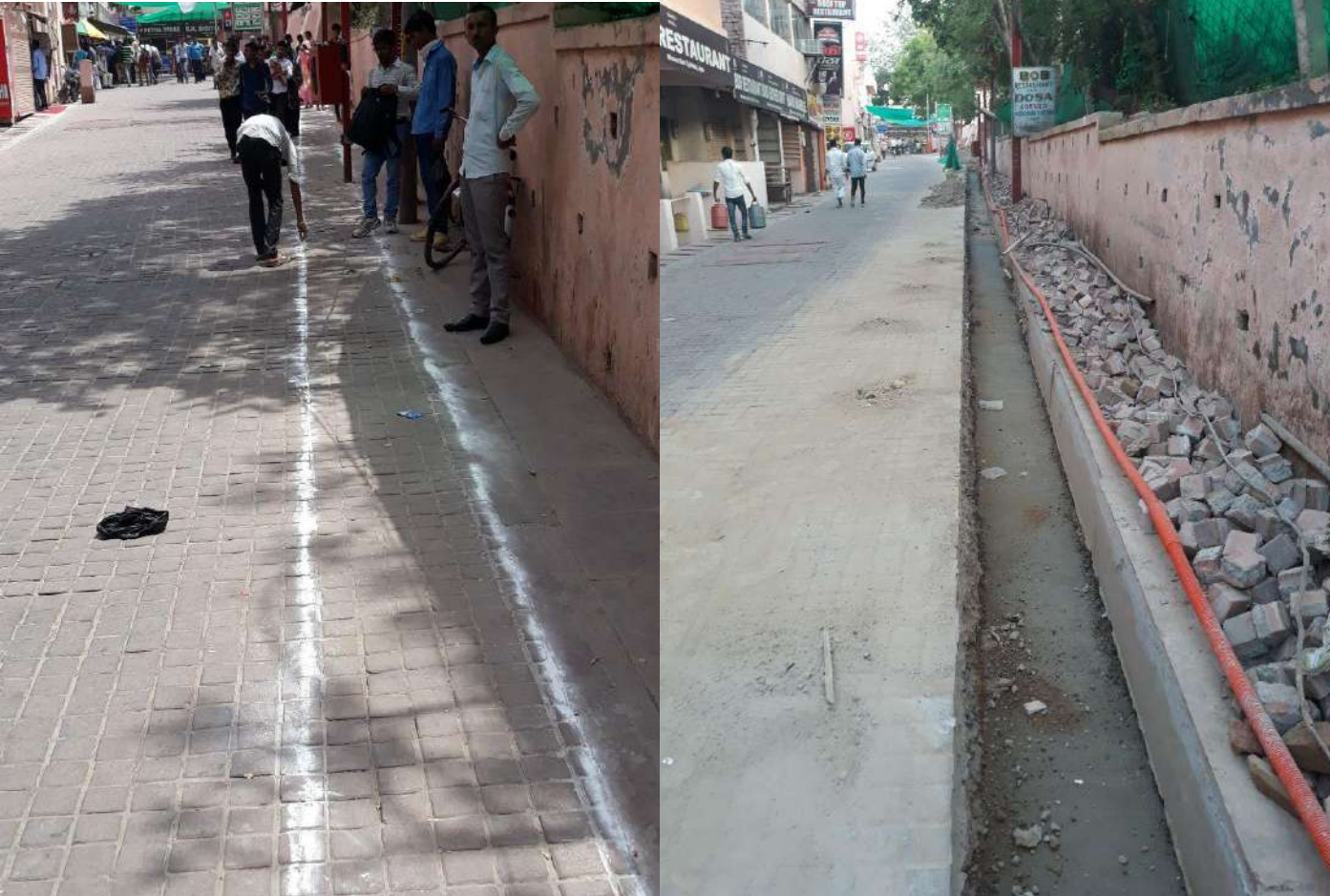
PCC for Utility done 80m
