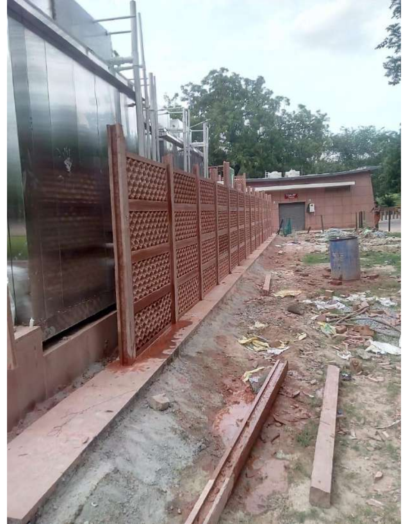
STONE JALI CLADDING ON E-TOILET NEAR TAJ WEST GATE
