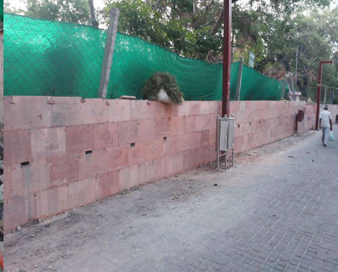
Stone Veneer work done 70m
