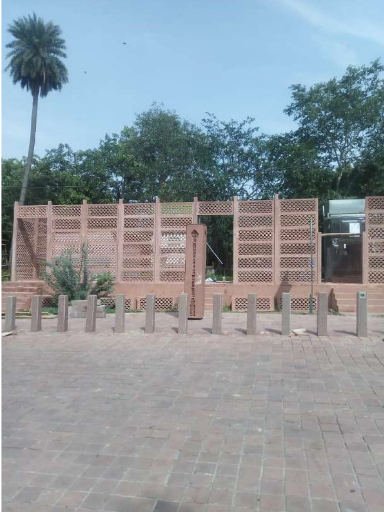
STONE JALI CLADDING ON E-TOILET NEAR TAJ WEST GATE
