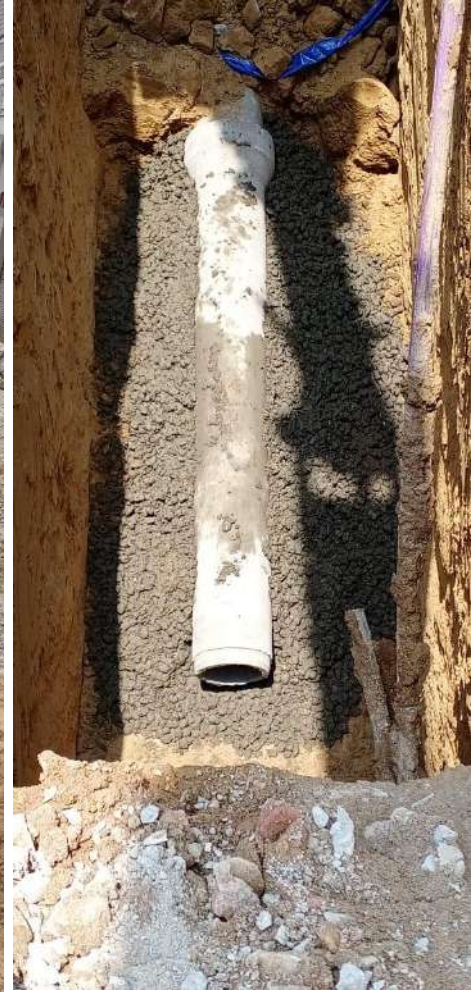
RCC 200 DIA PIPE LAYING
