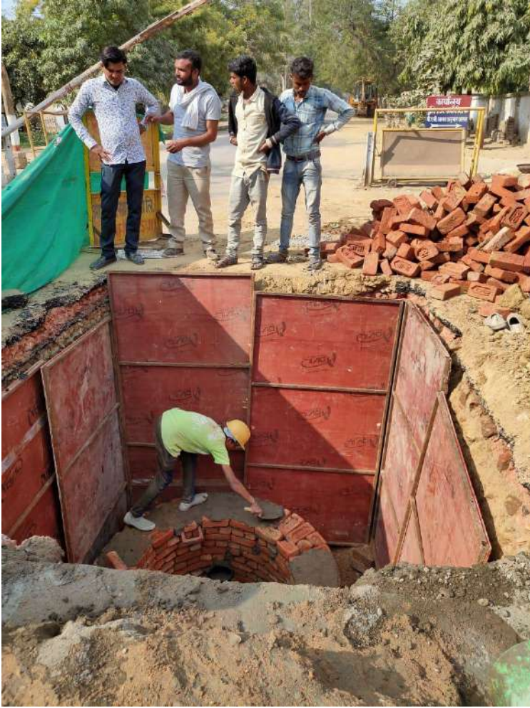
CONSTRUCTION OF MANHOLES
