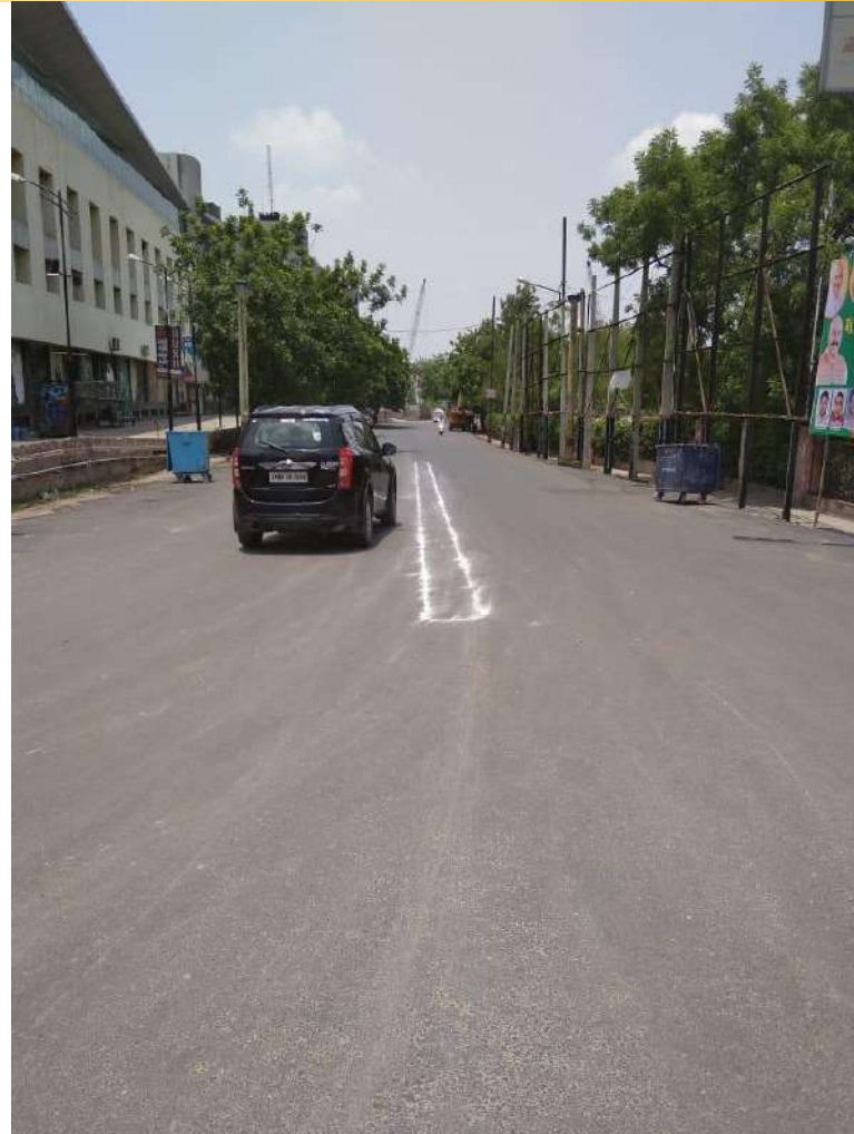
Coordinate Markings and Point Marking at Site
