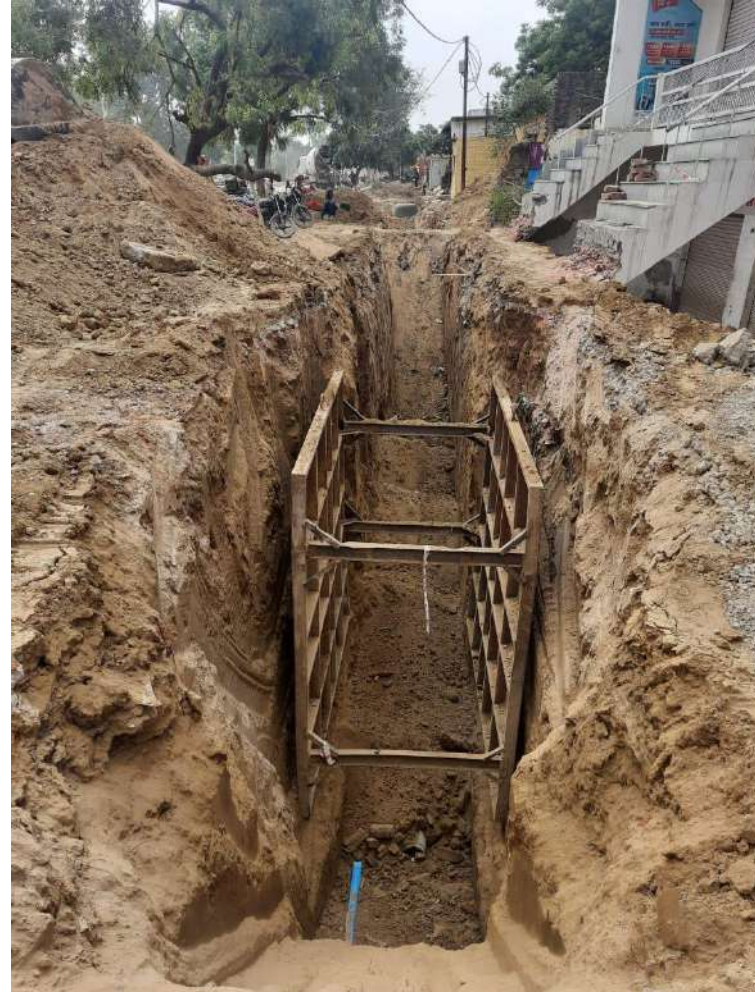
STEEL SHORING NEAR
