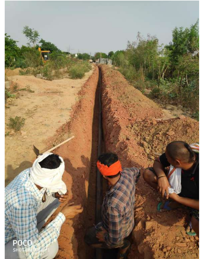
LAYING OF DISTRIBUTION NETWORK
