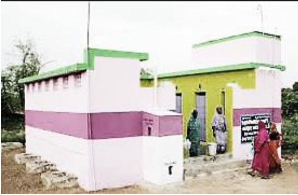
Typical Sanitary/ Toilet Complex
