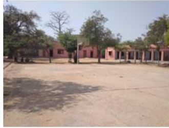
Cracks in basketball court
