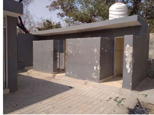
No shaded passage for approaching toilets
