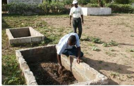
Decomposing waste pit
