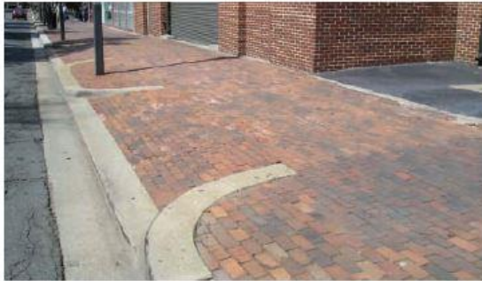
Driveway designed as a curb cut, not a minor junction, Washington, USA.
