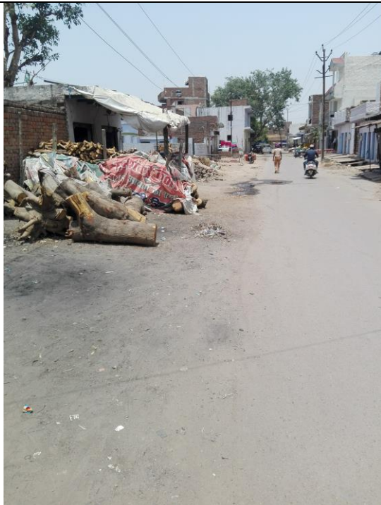
Left side-Chainage 520m to 670m The drain cross from left to right
