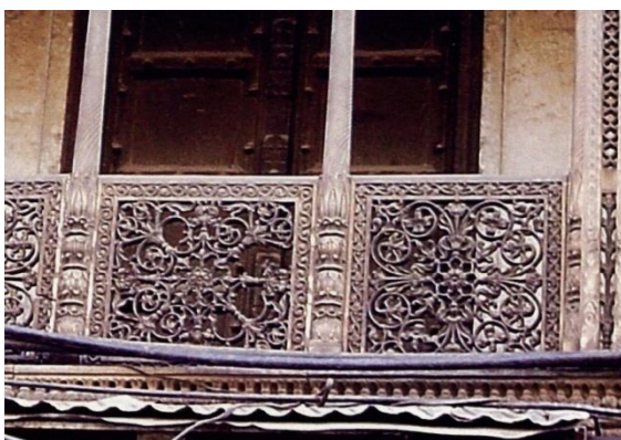
Figure 18: Ornate Wrought Iron and stone jali patterns in railings. Old wooden doors seen in backdrop.
