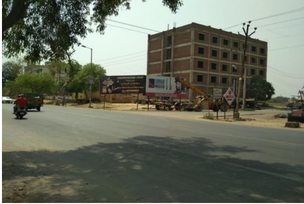
Zonal Park TajNagri Phase 2 crossing
