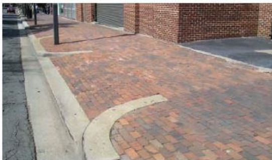
Driveway designed as a curb cut, not a minor junction, Washington, USA.
