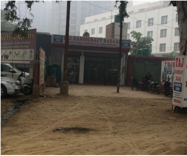
No Storm Water Drain
