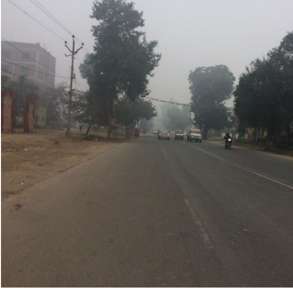
No Median available some of the portion
