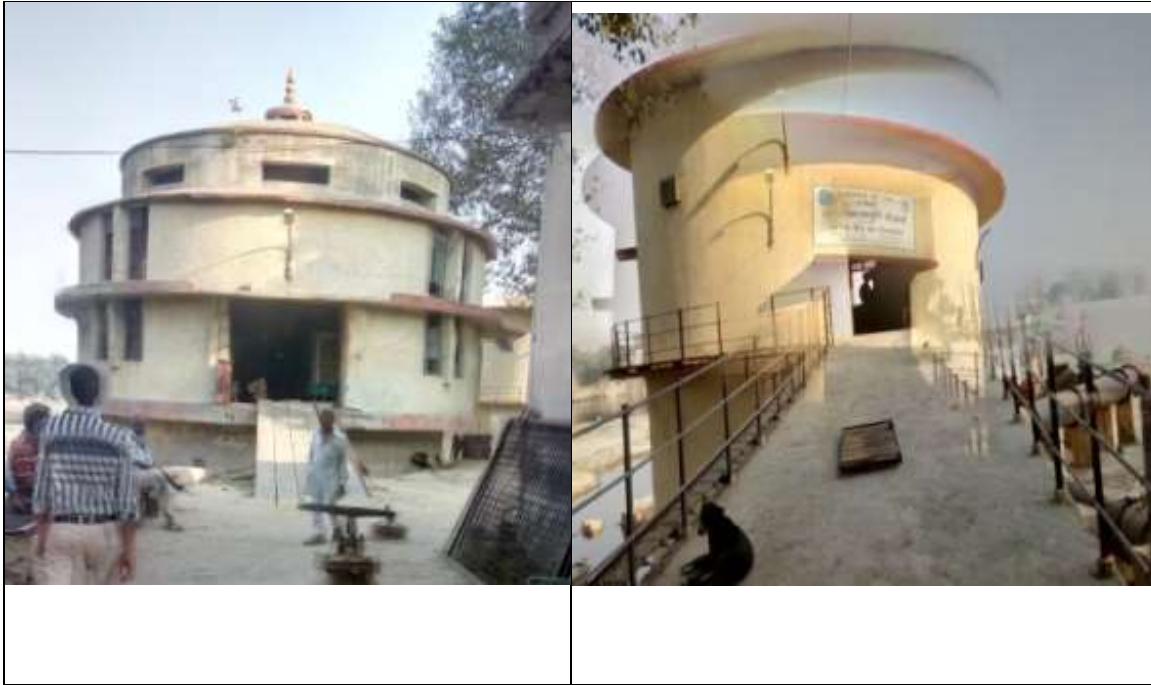
Figure 2: Intake works at JeoniMandi Water Works
