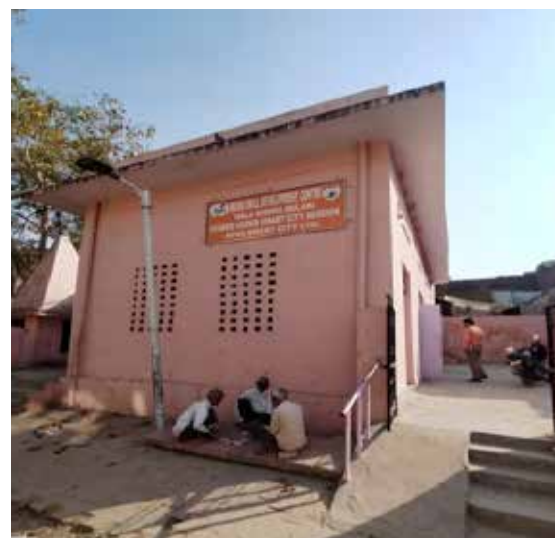
Figure 5: Entrance to Micro Skill Development Centre at Nala Shekh Bulaki. Source: Authors
